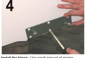
**Install the hinge:** Use small amount of marine sealant in each hole. Do not use excessive force when installing screws - ream the hole if necessary.
